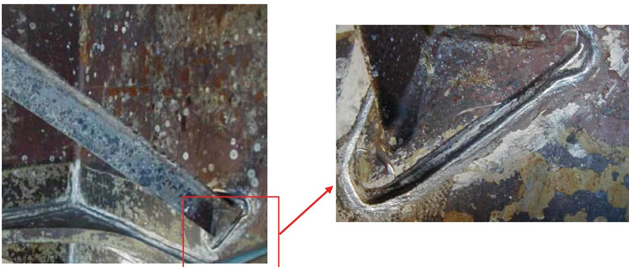
Figure 13.70 – Attachment for cable ladder inside brace: toe ground and needle peened.
