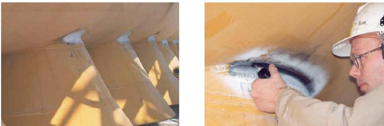
**Figure 13.72 – a) Bellmouths with highly stressed regions that have been examined by magnetic particle inspection (MPI) in preparation for weld improvement by grinding and needle peening and b) needle peening of bellmouth weld.**
