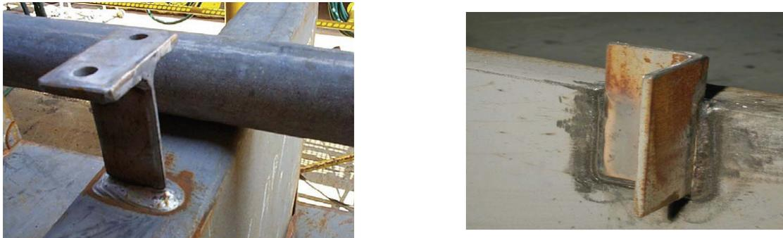
Figure 13.73 – Pipe attachments, flat bar welded to top of beam and angle profile welded to side of beam.
